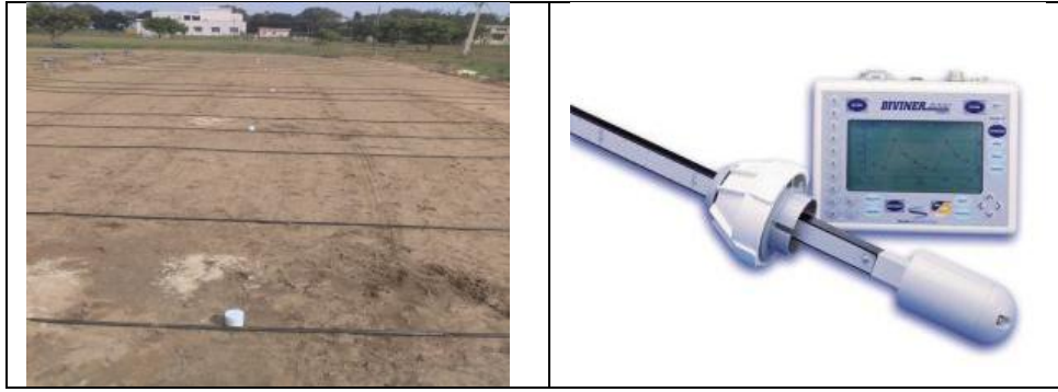
Plate 2 Installed access tubes and FDR sensor
