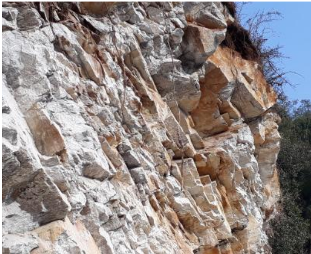
Plate 1. A Fragile Rock Structure
