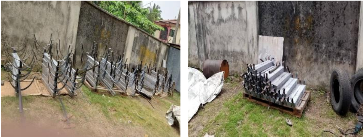
Fig. 2. Images of the fabrication of the anode-clamp assembly
