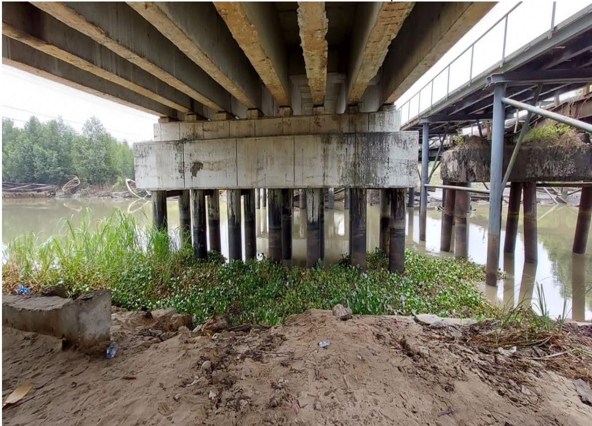
Fig. 1. Image of the 60 m reinforced concrete bridge structure
