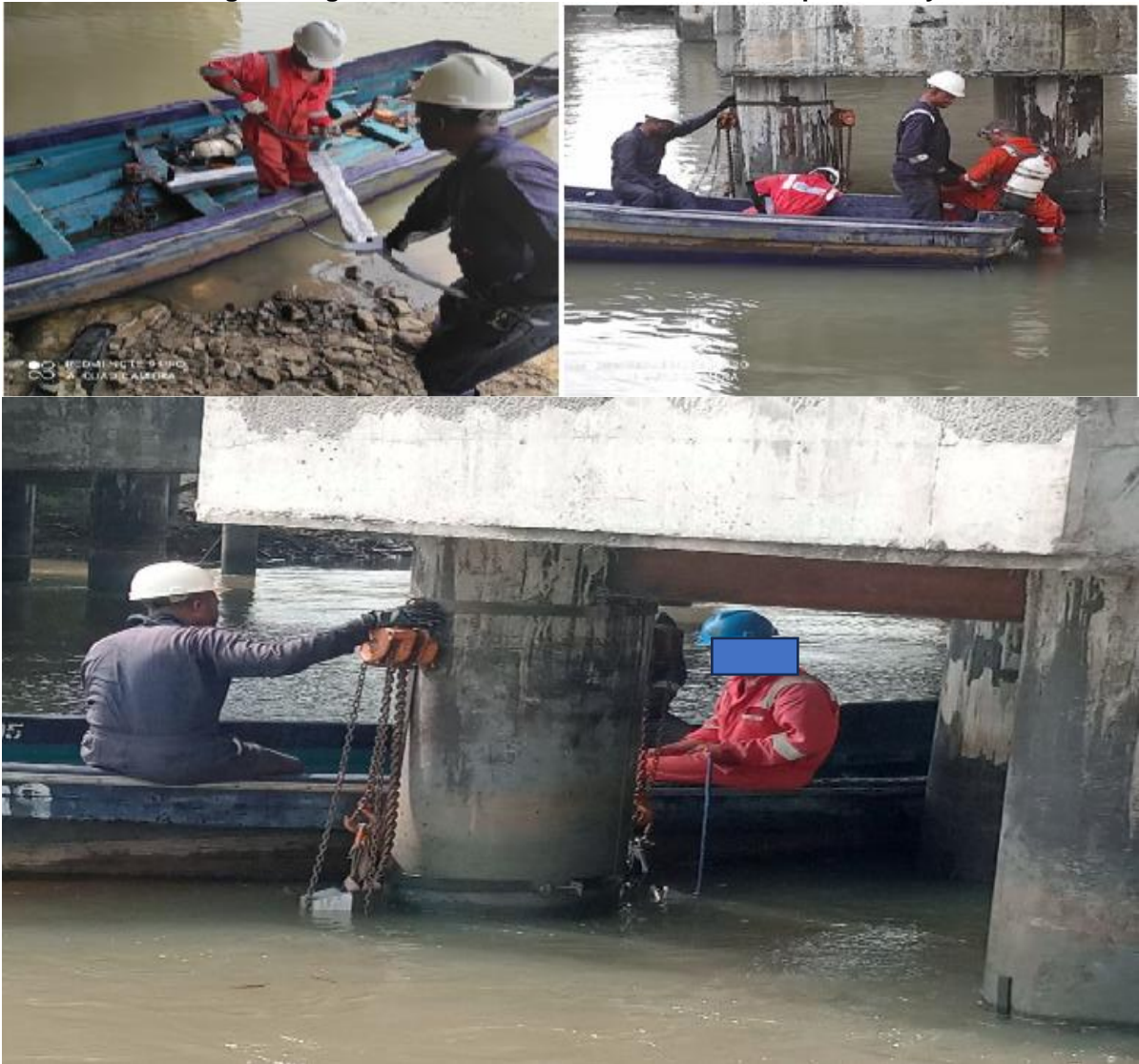
Fig. 3. Images of the installation exercises of the galvanic anodes
