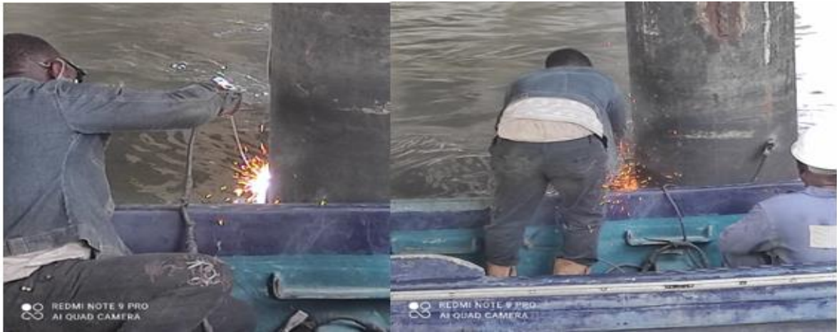
Fig. 4. Images of welding exercise of the anodes on the casing pipes
