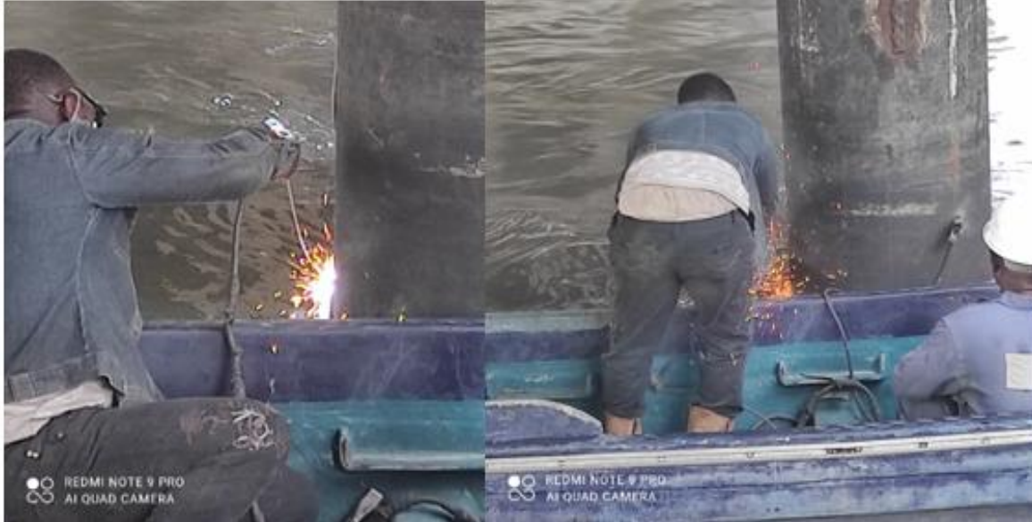
Fig. 4. Images of welding exercise of the anodes on the casing pipes
