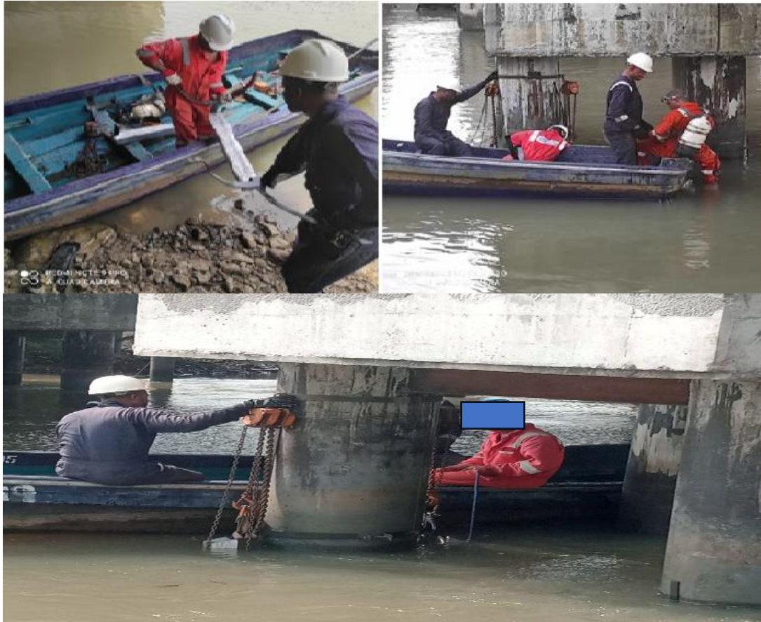
Fig. 3. Images of the installation exercises of the galvanic anodes
