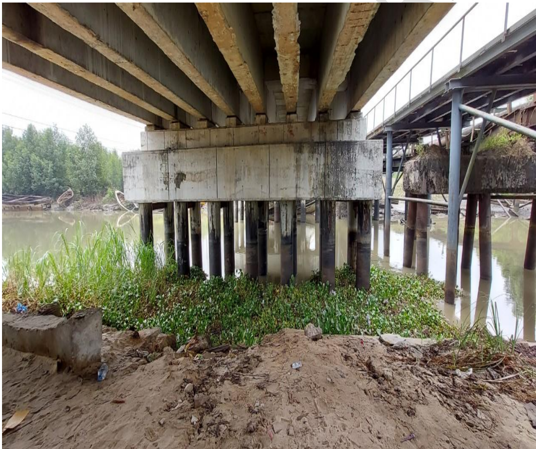
Fig. 1. Image of the 60 m reinforced concrete bridge structure
