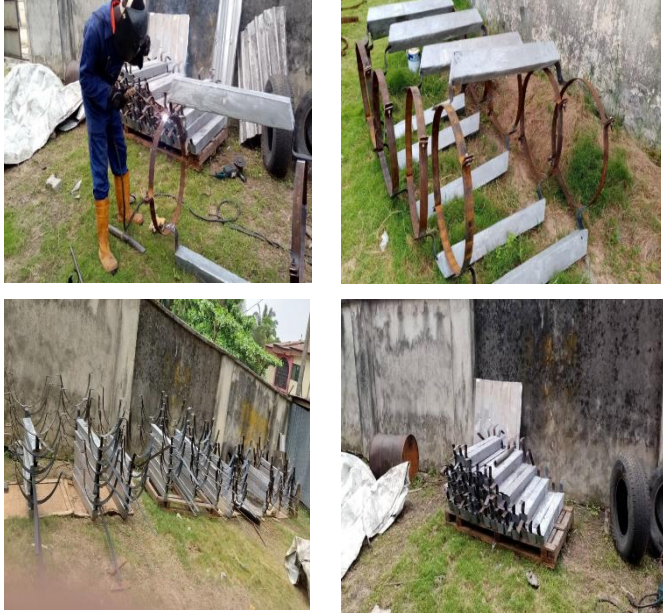
Fig. 2. Images of the fabrication of the anode-clamp assembly
