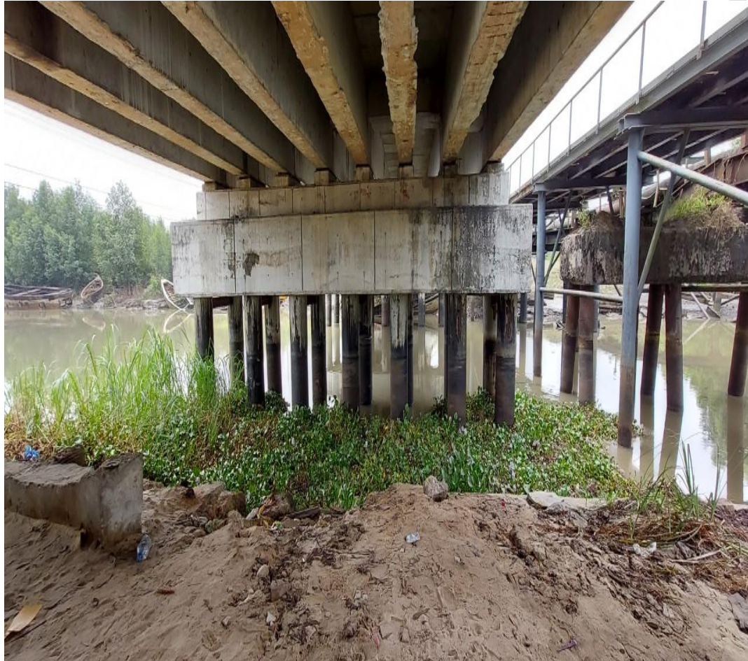
Fig. 1. Image of the 60 m reinforced concrete bridge structure
