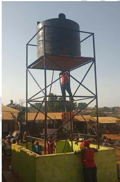
Village borehole in a market square
