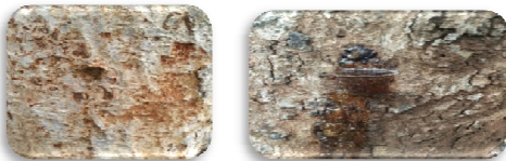
Covering with clay
