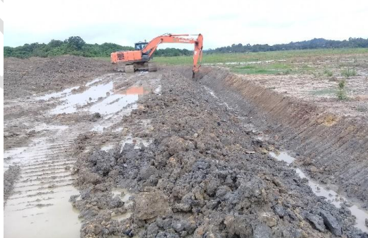
Figure 4. Construction of Erosion Control Channels
