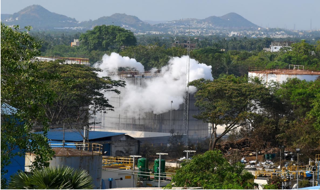
Fig.3.A file photo of styrene gas leaking out of a tank in LG Polymers unit, in Visakhapatnam
