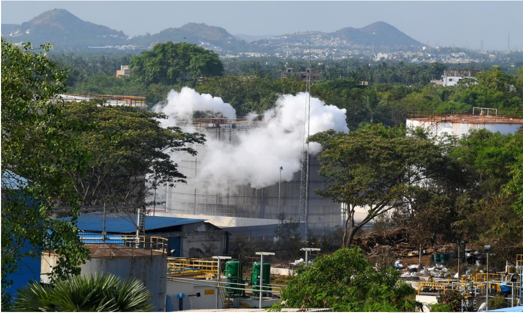
Fig.3.A file photo of styrene gas leaking out of a tank in LG Polymers unit, in Visakhapatnam
