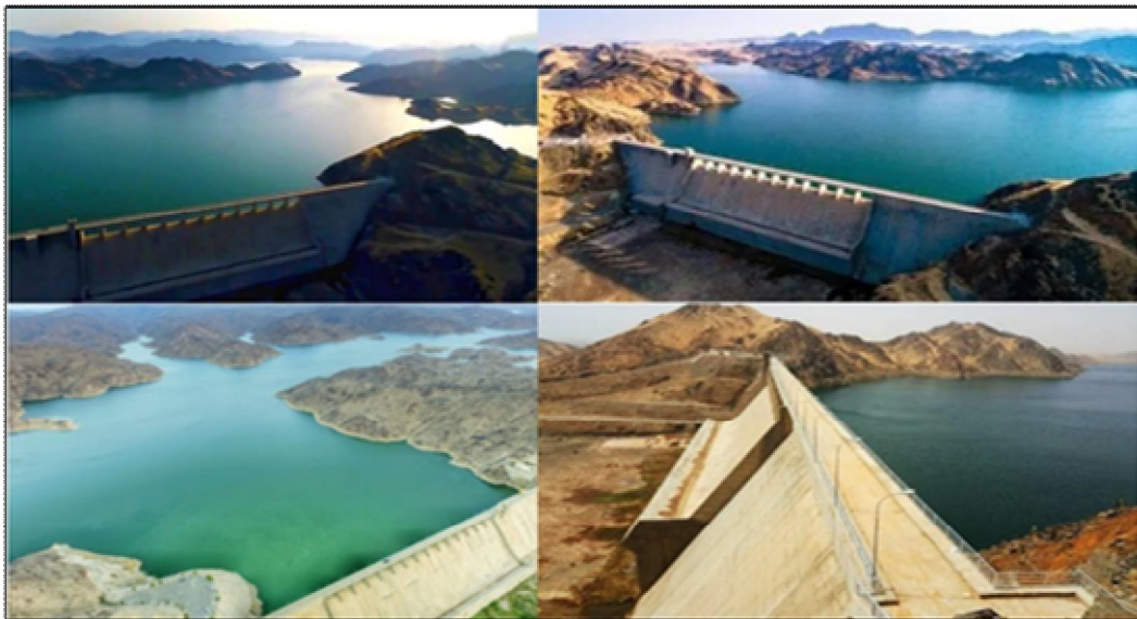
Figure 1: Shows the Major two dams in Kingdom of the Saudi Arabia.
