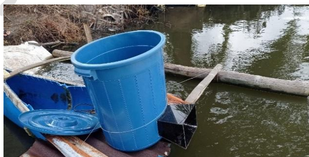
Figure 16. Actual Set-up of the Project
