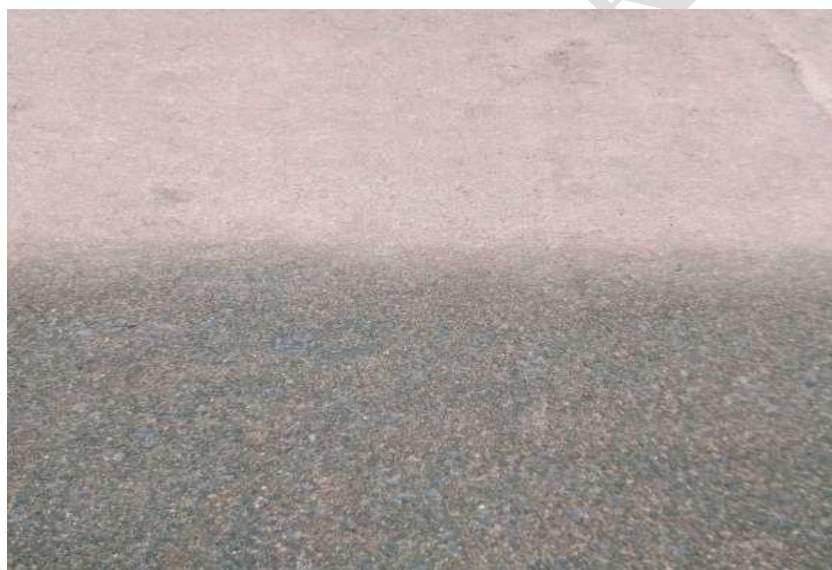
Figure 3: Observation of Concrete Face Above and Below the Free Board
