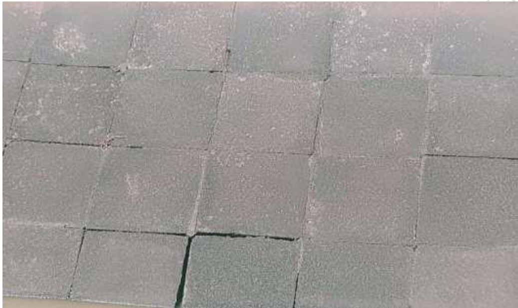
Figure 8: Removal of Joints between the Joints of Precast Concrete
