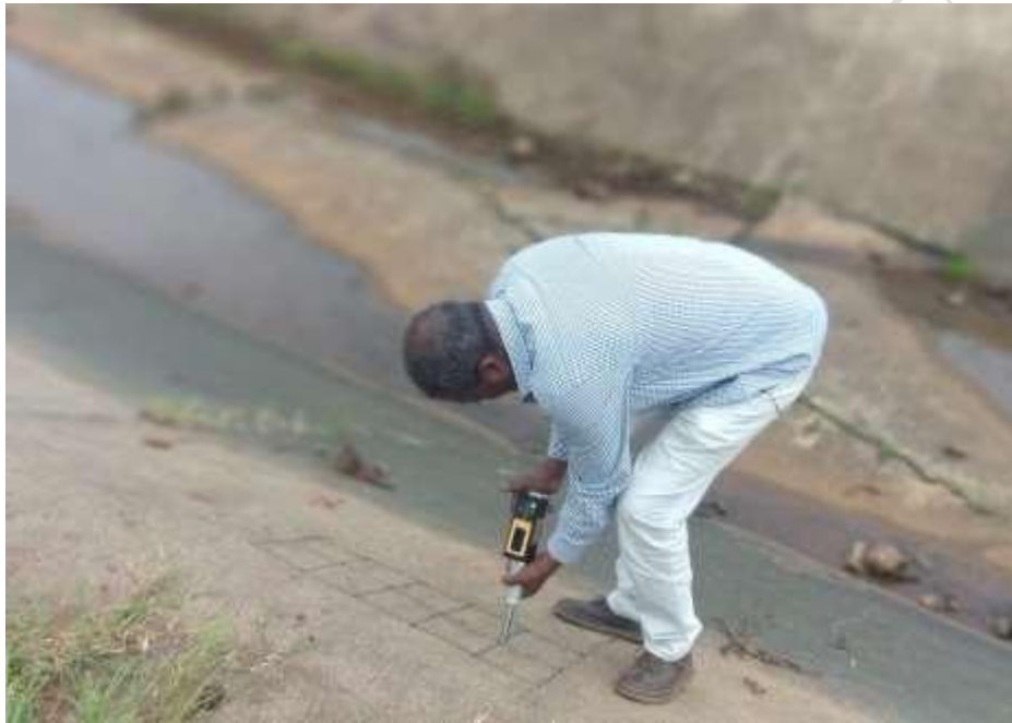
Figure 9: Conducting Rebound Hammer Test
