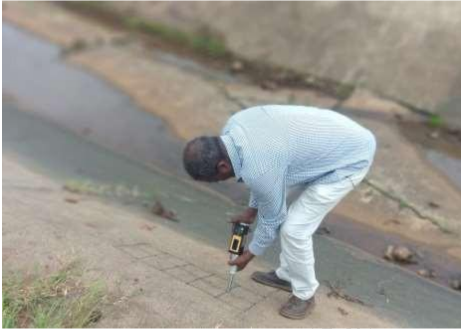
Figure 9: Conducting Rebound Hammer Test
