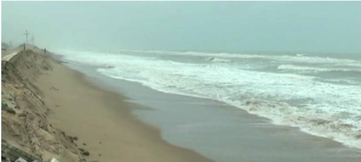
Fig 6: Coastal erosion near Rama Chandi-Konark Road after the great Indian Tsunami 2004.
