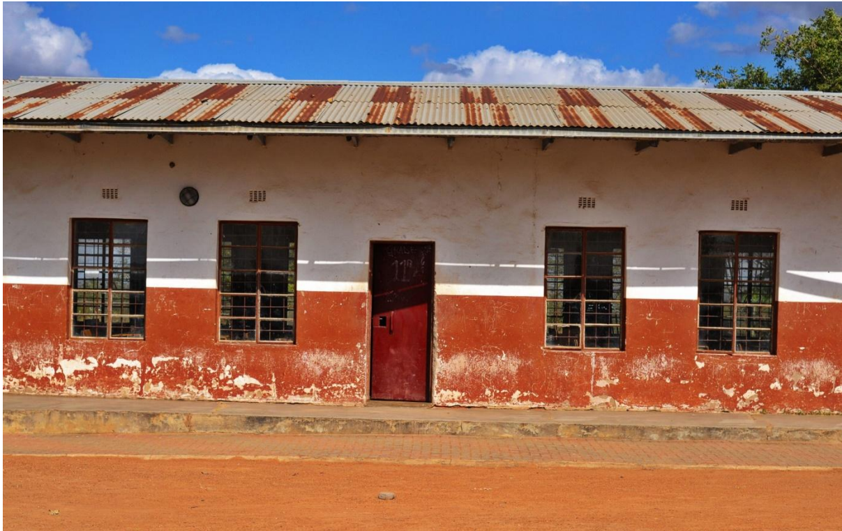
Fig 2. Netshimbupfe Secondary School
