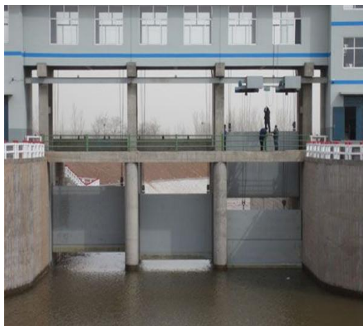
Fig. 1 Flat steel gates application in practical engineering
