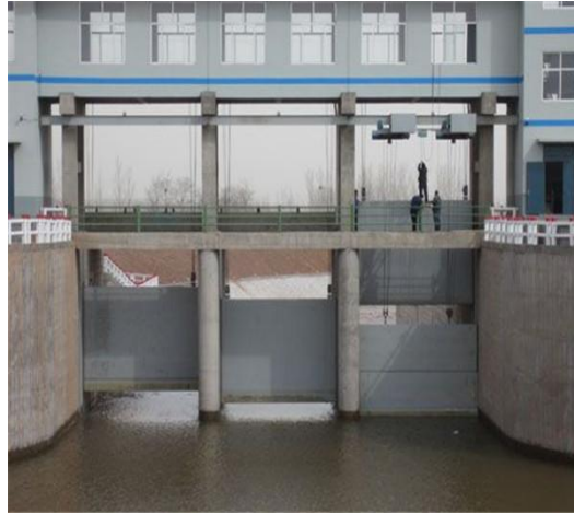
Fig. 1 Flat steel gates application in practical engineering
