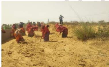
Land Development work in Rajasthan
