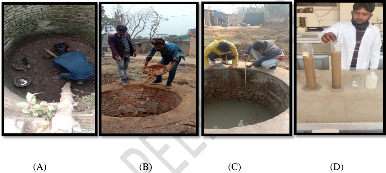
Picture1 : Drywell recharge work in selected sites of District Ambedkarnagar
