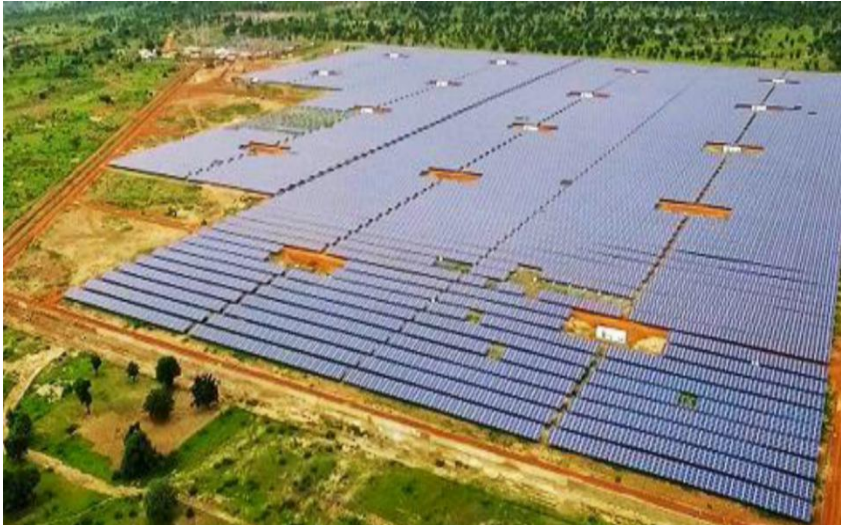
Figure 1 : Aerial view of the Zagtouli solar power plant.
