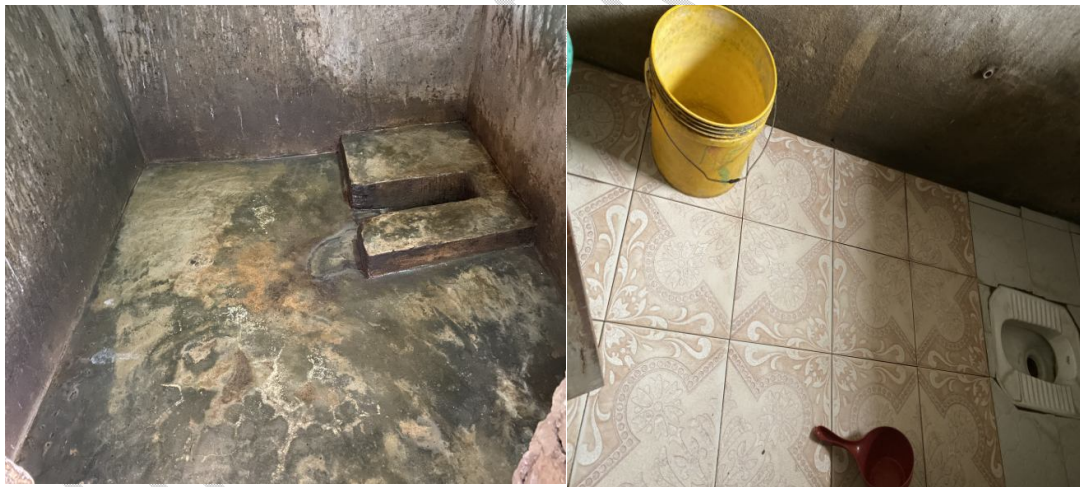
Figure 2: Latrine types available; a) Open pit b) Dry pit
