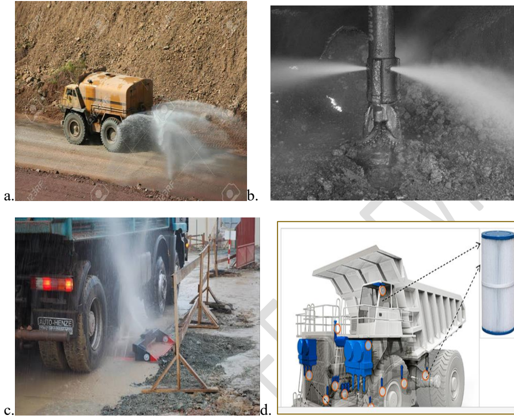
Fig 20 (a-d): - Water sprinkling method on the road(b) Wet drilling method (c) Wheel wash technique (d)- HEPA Filter in heavy vehicles
