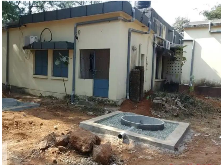
Fig 21: Rooftop rainwater harvesting in the block office at Sukinda Block office
