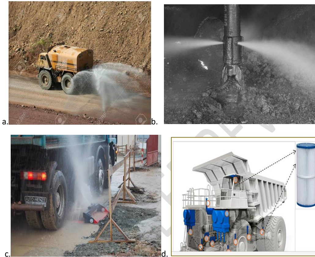
Fig 19 (a-d): - Water sprinkling method on the road(b) Wet drilling method (c) Wheel wash technique (d)- HEPA Filter in heavy vehicles
