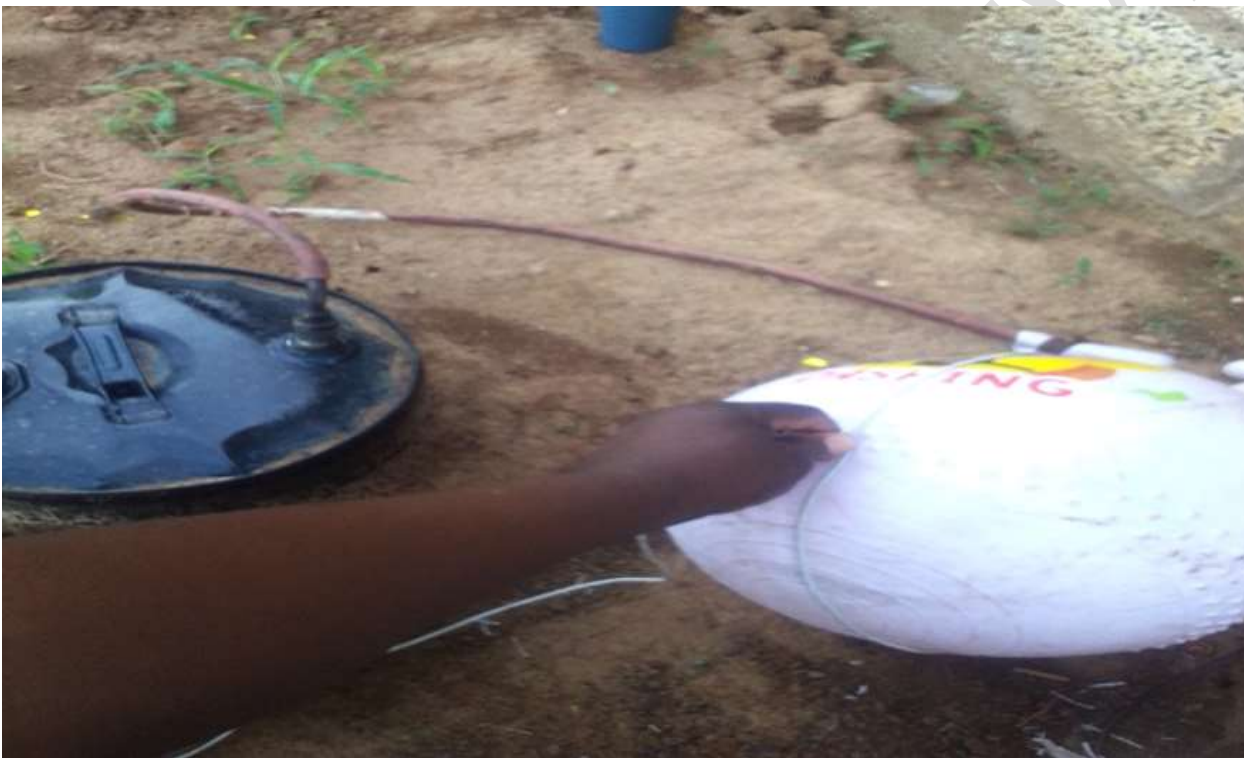
Figure 5. Shows a Metallic Drum Bio digester and a balloon as biogas collection chamber
