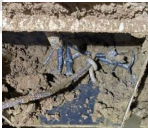
Fig. 8. difficulty in discharging slag
