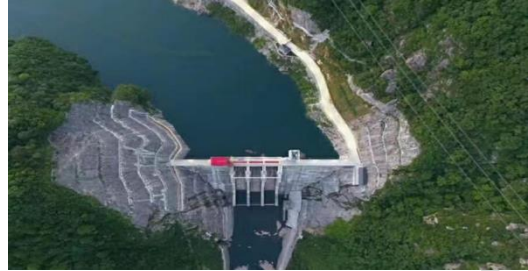
Fig. 4. Hongping pumped storage power station
