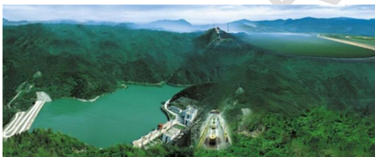
Fig. 2. pumped storage power station
