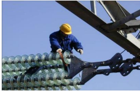
Fig.5. Hanging insulator string horizontally
