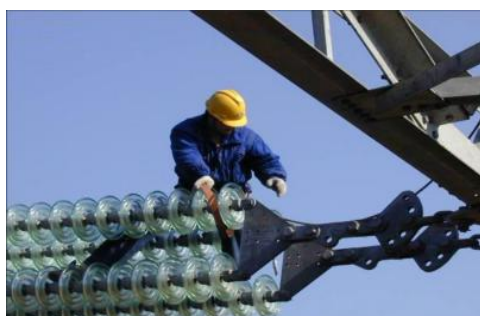
Fig.5. Hanging insulator string horizontally
