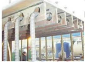
(b) Steel-concrete bonding section-PBL.
