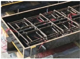
(a) Steel-concrete combination beams-PBL.
