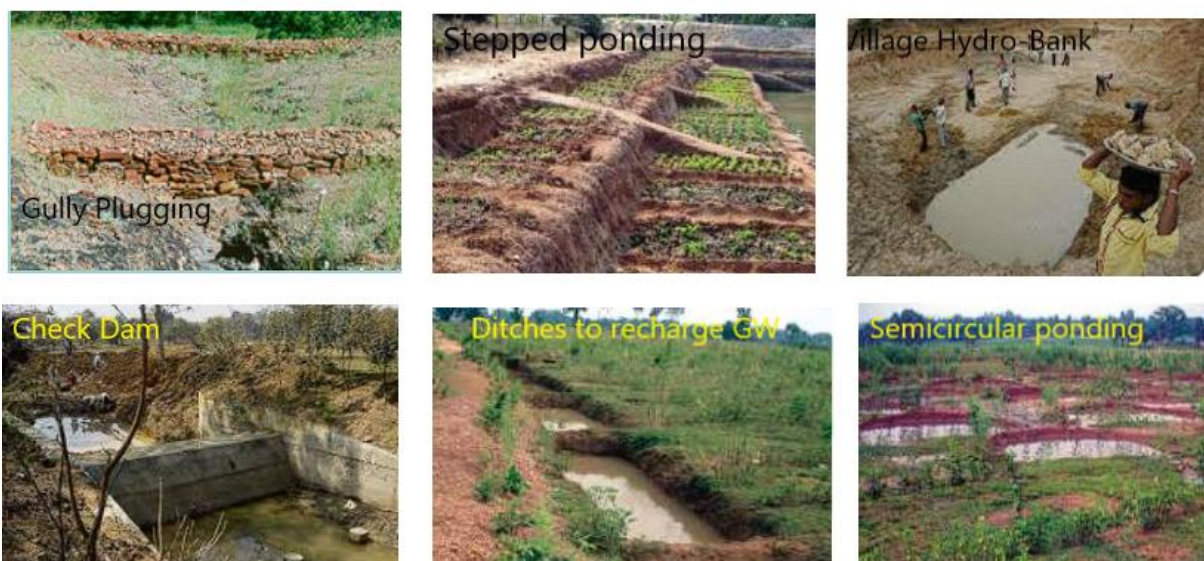
Fig.10. Some water harvesting structures and groundwater recharging units to combat drought
