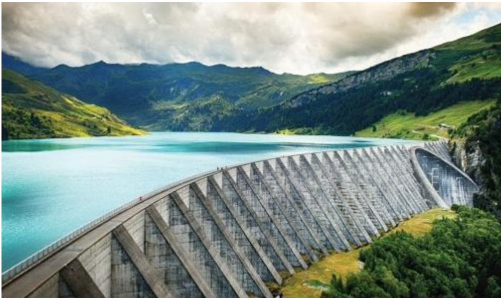
Figure 15: Roselend Dam, Beaufort, France (source: IRENA, 2018)
