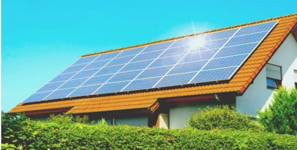
Figure 13: Roof-mounted Solar panels (source: Stern, Burke and Bruns, 2019)
