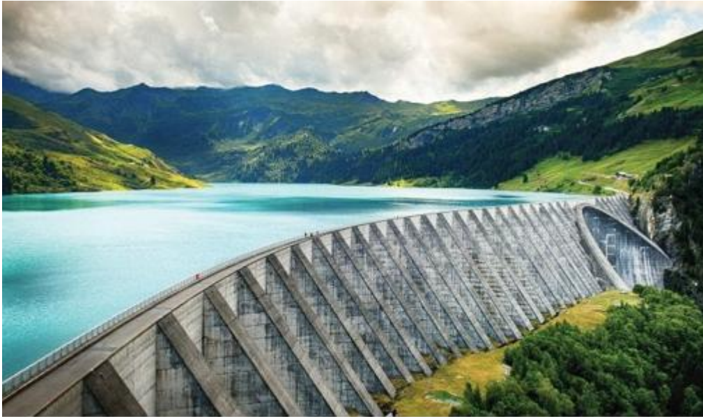
Figure 4: Roselend Dam, Beaufort, France (source: IRENA, 2018)
