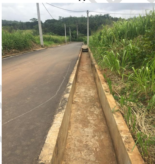
Figure 1: Delayed electricity, tarred road and drainage
