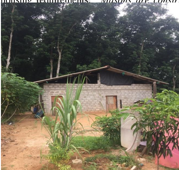
Figure 6: Half erected house with no funds in hand
