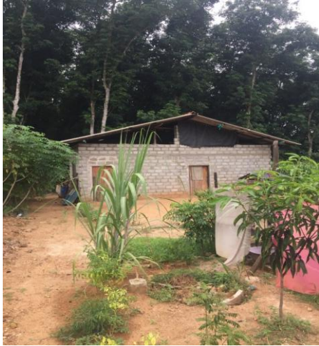
Figure 6: Half erected house with no funds in hand
