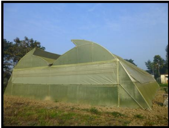
Plate 1: Showing site view
