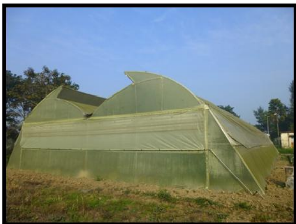
Plate 1: Showing site view
