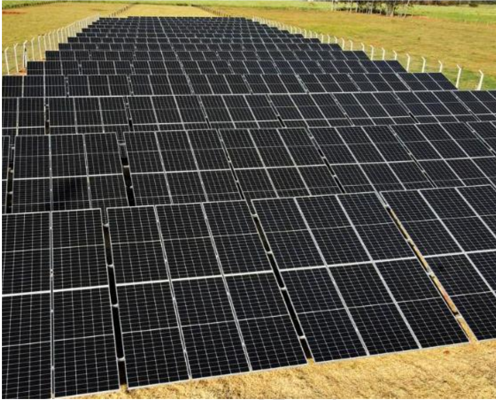
Figura 5. Instalation of the panel
