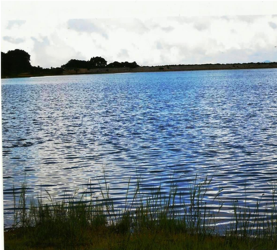
Plate II: The Wulmi River Passes through Pankshin Dam which serves as Reservoir for the Pollutants.
