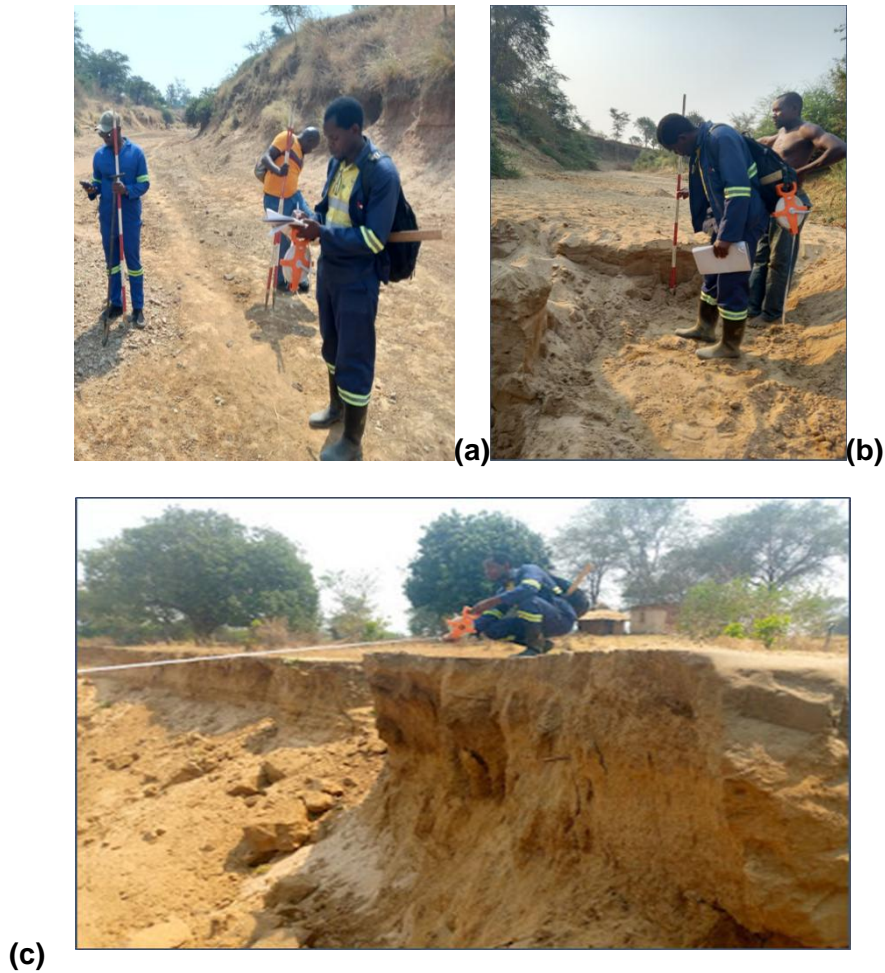
Fig 2: (a-b) Field measurements of sediment depth and (c) Degraded channel and bed morphology of the Magoye River.
