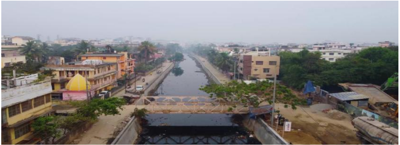
Figure 7: A major portion of the River Bharalu lacks vegetation of either side of its banks due to rapid urbanization and regular cleaning of this stretch to prevent flash flood.
