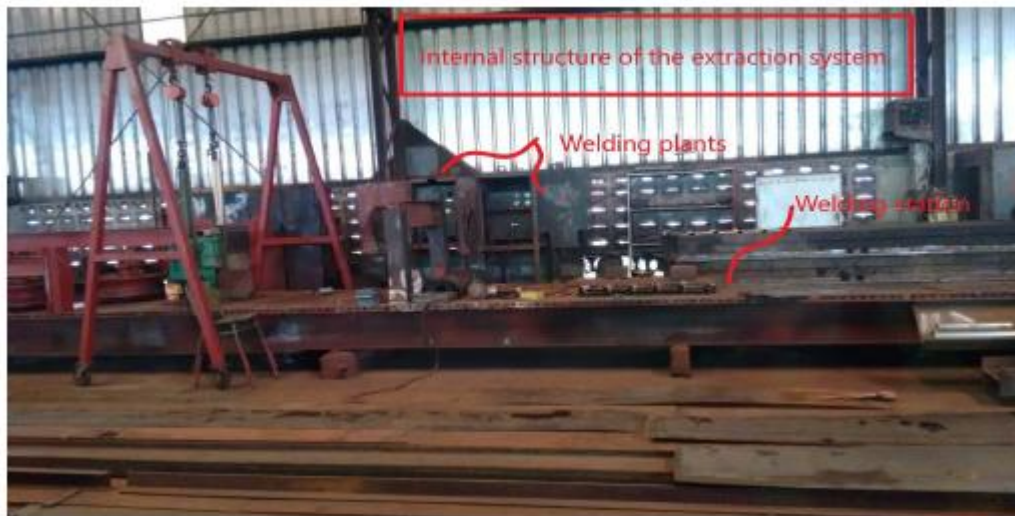
Fig. 2. Inside view of the extraction system and its easy access to the welding station
