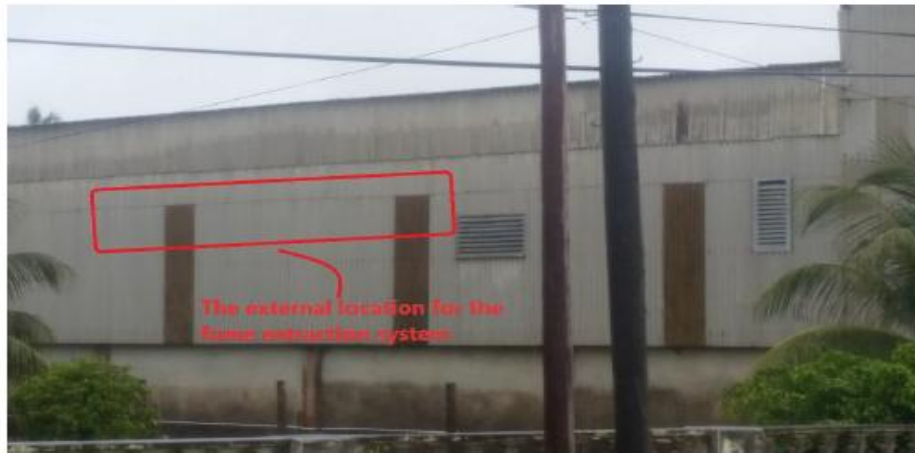
Fig. 1. Outside view where the extraction system will be mounted
