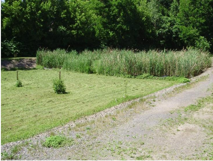
Fig 7: Subterranean Flow Constructed Wetland Cell 1 [31]
