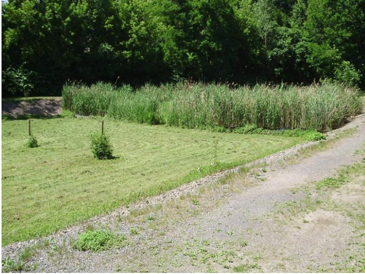
Fig 7: Subterranean Flow Constructed Wetland Cell 1 [31]
