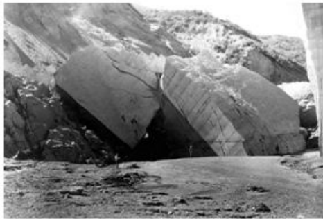
Figure 2 St. Francis Dam Break
