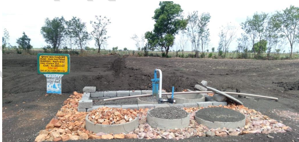
Fig. 1. A farm pond for Ground water/tube well recharge at IWMRC Belavatagi (before recharging Rain fall events )
