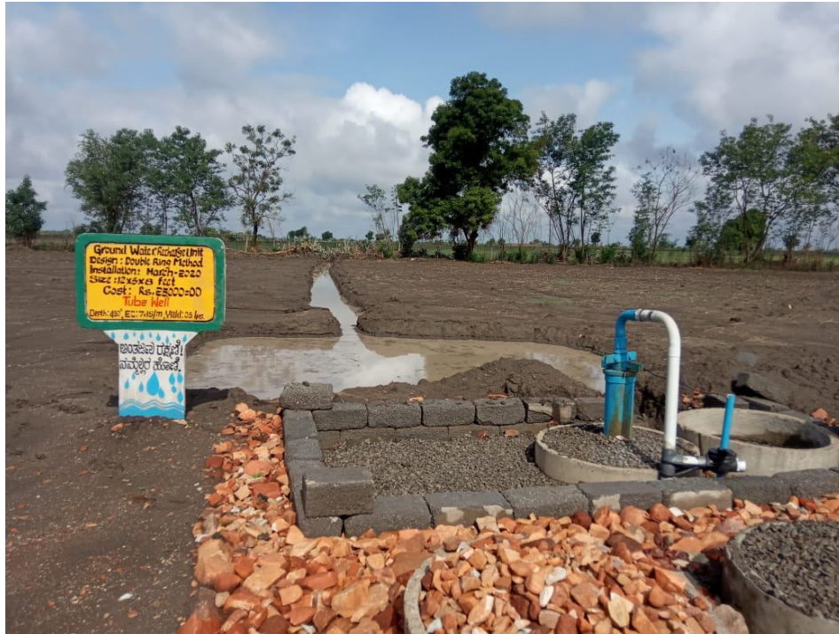
Fig. 2. A farm pond for tube well recharge at IWMRC Belavatagi (After recharging Rain fall events )
