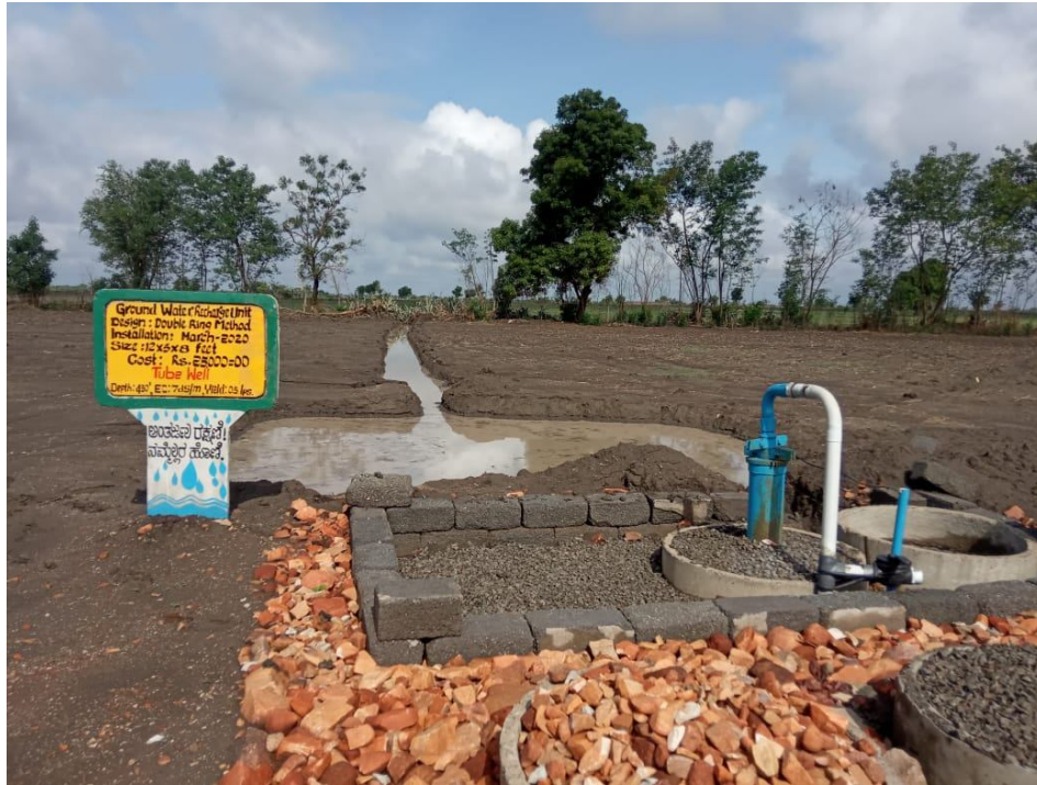
Fig. 2. A farm pond for tube well recharge at IWMRC Belavatagi (After recharging Rain fall events )
