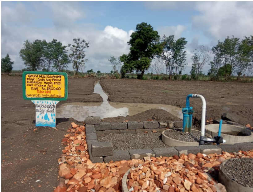
Fig. 2. A farm pond for tube well recharge at IWMRC Belavatagi (After recharging Rain fall events )
