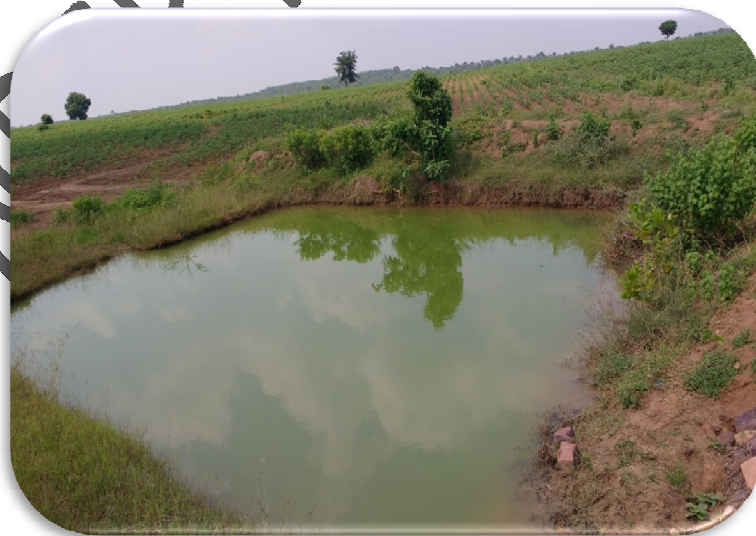
Plate 1 A view of a water harvesting structure
