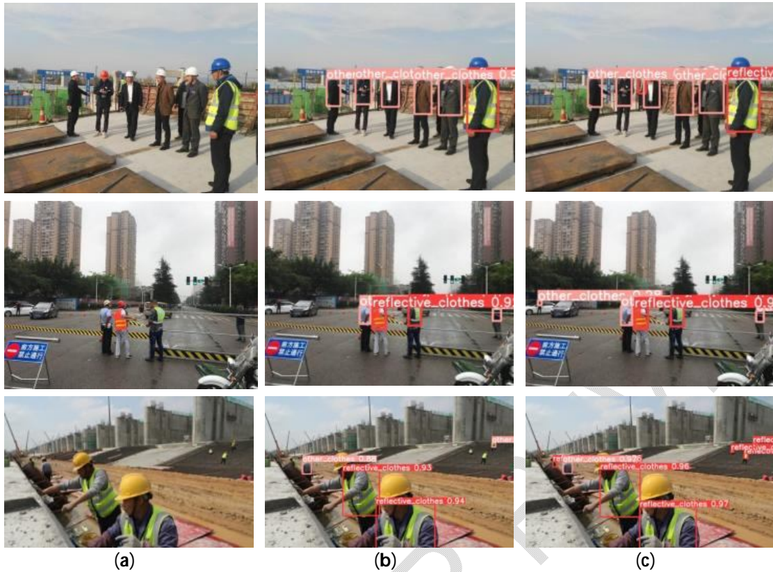
Fig. 8. Comparison of detection effects: (a) The original image; (b) Detection results based on YOLOv3; (c) Detection results of Yolov3 with CA mechanism
